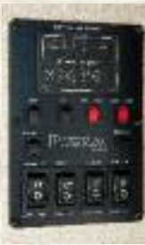
Switch panel controls slides, lights, porch light, water pump/heater; monitors battery and tank capacities
